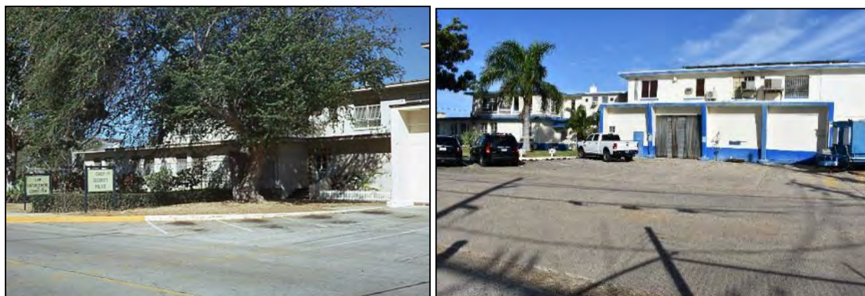
6 Building 406 (Fire Station): Photo 6.1-235, left, south front elevation in 1972-1973 (source: 7 https://rameyafb.wordpress.com/2010/11/13/pictures-of-ramey-afb-puerto-rico/ ); Photo 6.1-236, right, similar but 8 broader view of south elevation.
