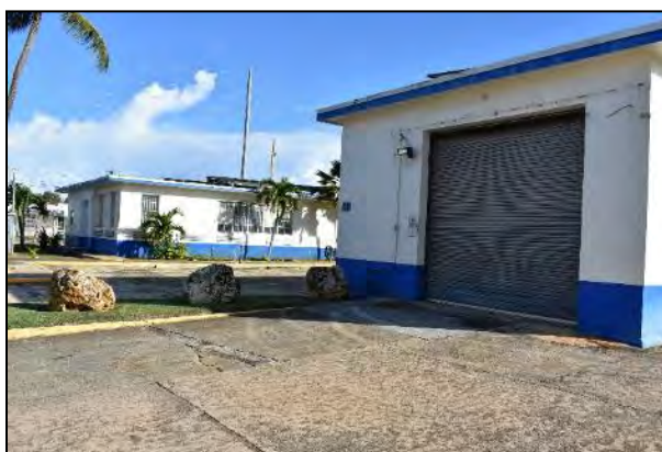
18 Photo 6.1-239, Building 407 (Paint, Oil, and Dope House): west front with Building 408 at left.
