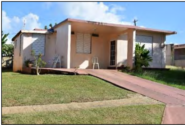
4 Photo 6.1-116 112 Loop Street
