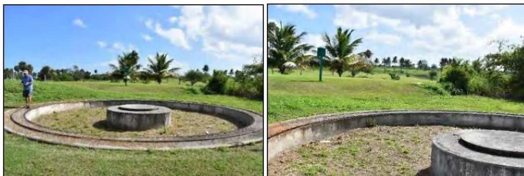
11 Photos 6.1-8 (left) and 6.1-9 (right) Southernmost Panama mount emplacement (Gerry Giles at far left).
