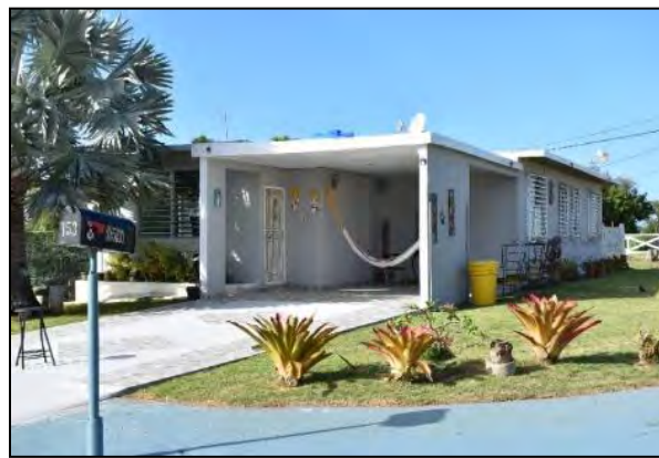
3 Photo 6.1-109 153 Lighthouse Drive
