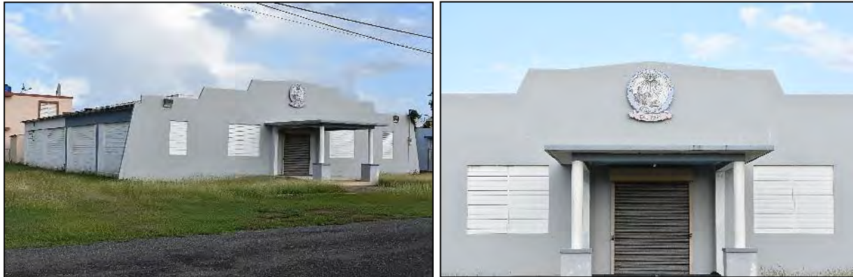
2 Paul Revere Lodge No. 98: Photo 6.1-501, left, north side and west front elevations showing edges of parapet front; 3 Photo 6.1-502, right, west front elevation with shield added after Hurricane Maria.
