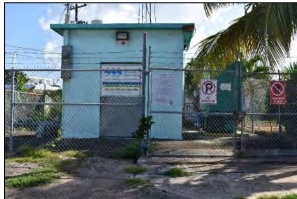
Photo 6.1-140 Utility building on lot between 130 Loop Street and 131 Lighthouse Drive
