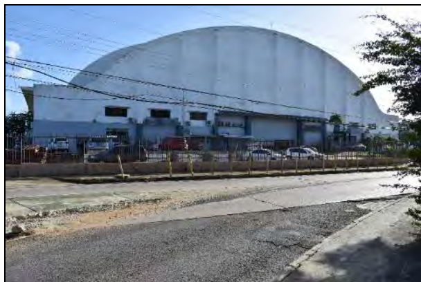
14 Hangar 3: Photo 6.1-282, left, north street-side elevation; Photo 6.1-283, right, north street-side elevations, note ribs 15 and infill of original hangar doors.
