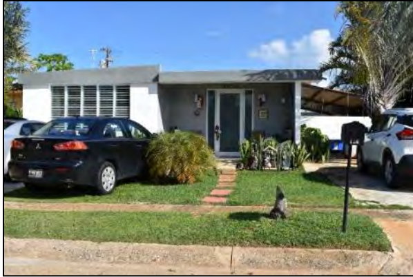
1 Photo 6.1-130 126 Loop Street
