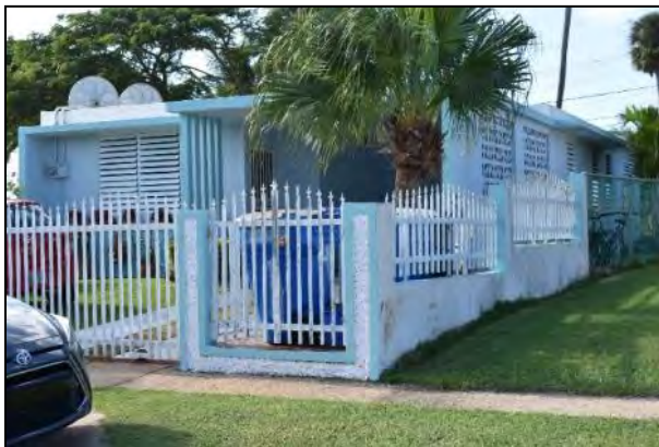
2 Photo 6.1-103 143 Lighthouse Drive
