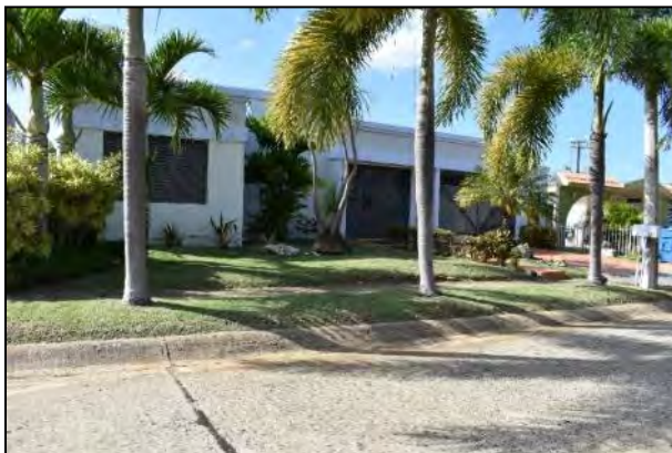
3 Photo 6.1-87 127 Lighthouse Drive
