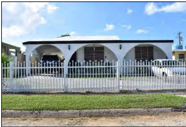
3 Photo 6.1-81 121 Lighthouse Drive
