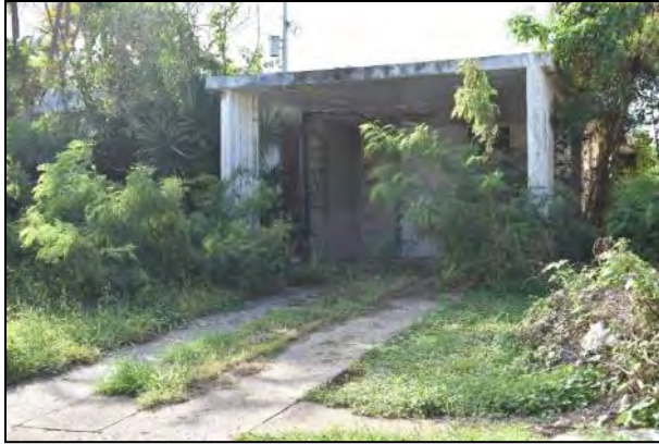
1 Photo 6.1-95 135 Lighthouse Drive
