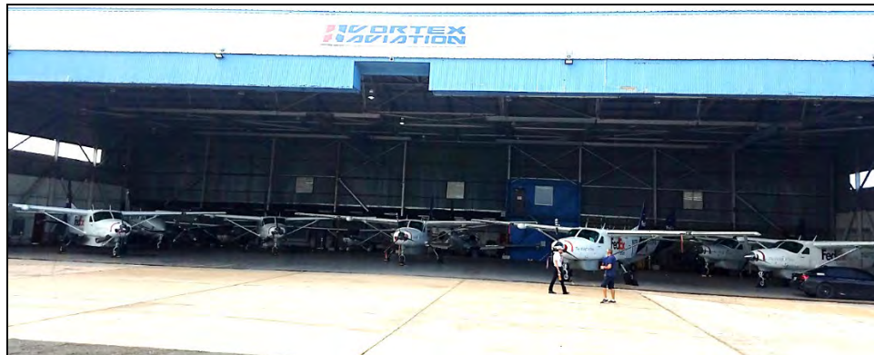
1 Photo 6.1-450 Building 573 (Nose Dock Hangar): south elevation and interior depicting retention of central notch for B- 2 52 tail, enclosure of nose dock, and addition of window bands at side elevations (source: Vortex Aviation website).
