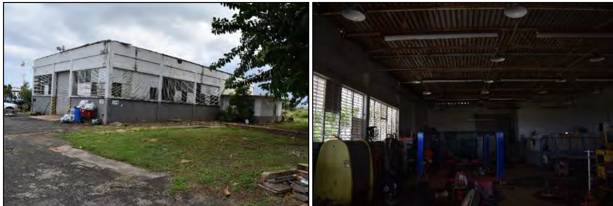
1 Building 1029 (Ground Support Equipment Shop): Photo 6.1-410, left, north rear and west side elevations; 2 Photo 6.1-411, right, interior looking north through rear louvers.
