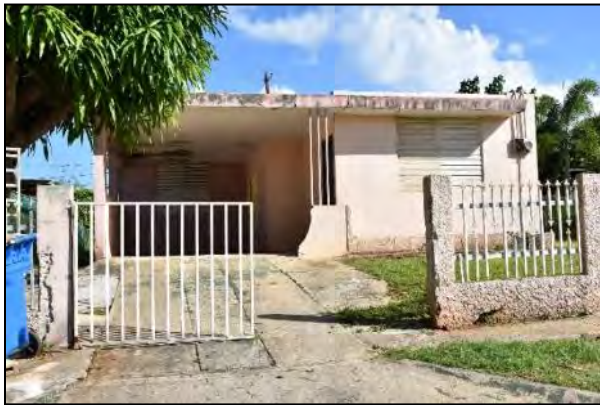
2 Photo 6.1-114 110 Loop Street
