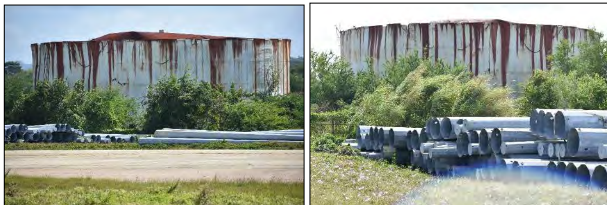
14 Tank 1215 (Fuel Storage Tank): Photo 6.1-476, left, looking south at tank, left to right; Photo 6.1-477, right, looking 15 southeast at tank.
