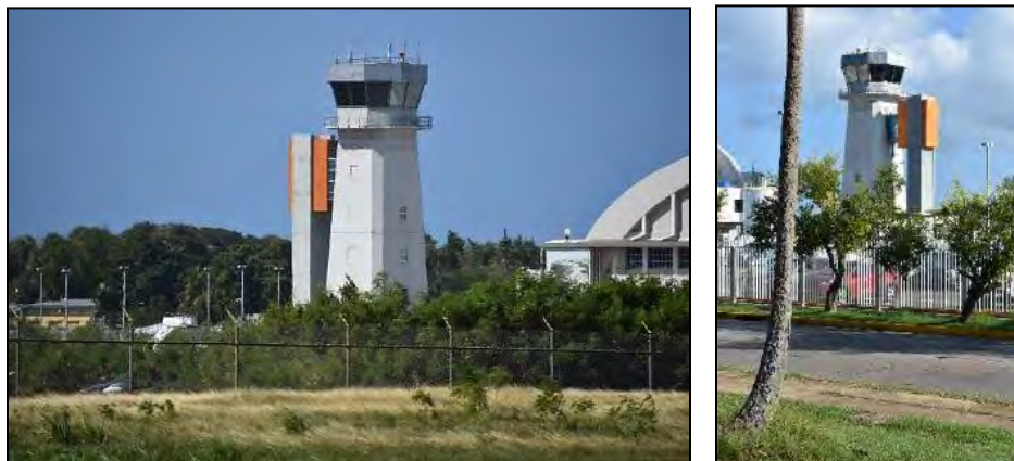
1 Control Tower: Photo 6.1-306 views looking northwest; Photo 6.1-307 looking southwest
