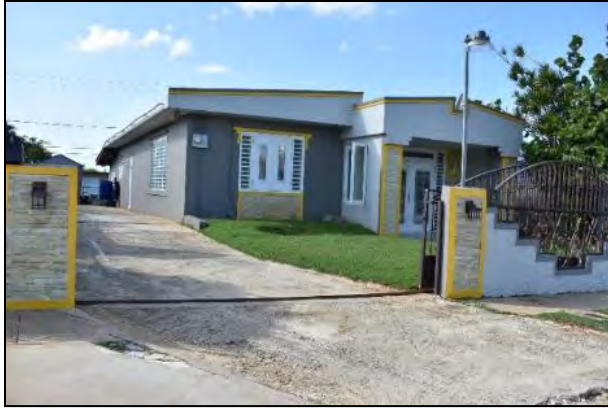
1 Photo 6.1-71 111 Lighthouse Drive
