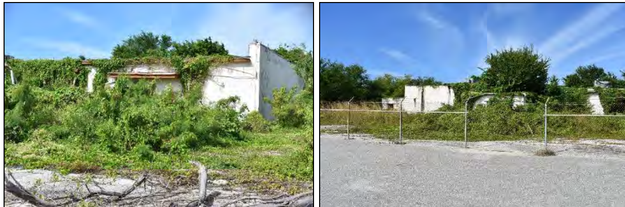
1 Building 1128 (Armaments and Avionics Shop): Photo 6.1-376, left, south front and east side elevations; right, south 2 front elevation.
