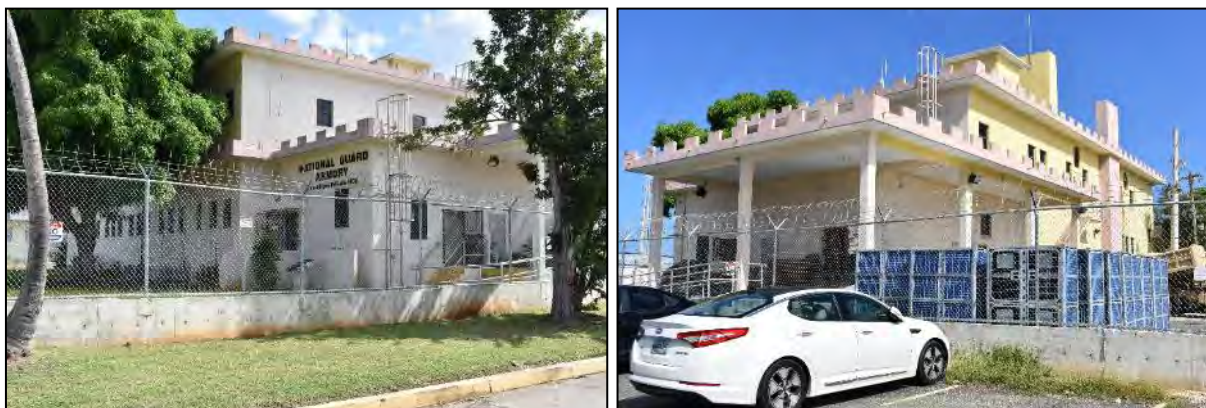
9 Building 504 (Bakery): Photo 6.1-193, left, north front and west side elevations: Photo 6.1-194, right, west side and 10 south rear elevations.
