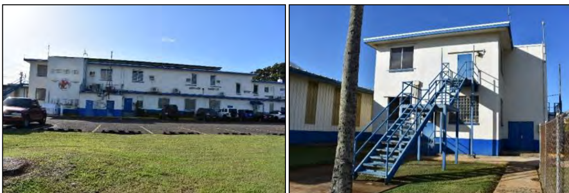
5 Building 406 (Fire Station): Photo 6.1-233, left, north rear elevation; Photo 6.1-234, right, east side elevation.
