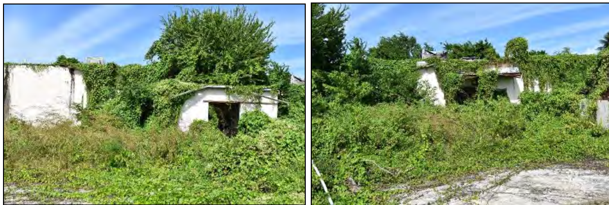
22 Building 1128 (Armaments and Avionics Shop): Photo 6.1-374, left, western third of S front elevation; Photo 6.1-375, 23 right, central third of S front elevation
