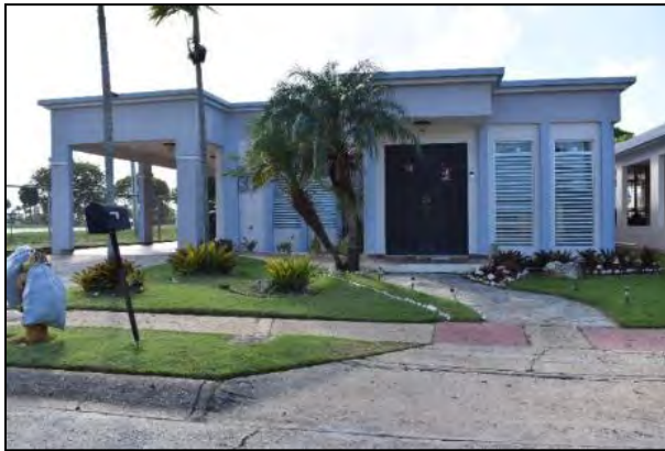
2 Photo 6.1-61 101 Lighthouse Drive
