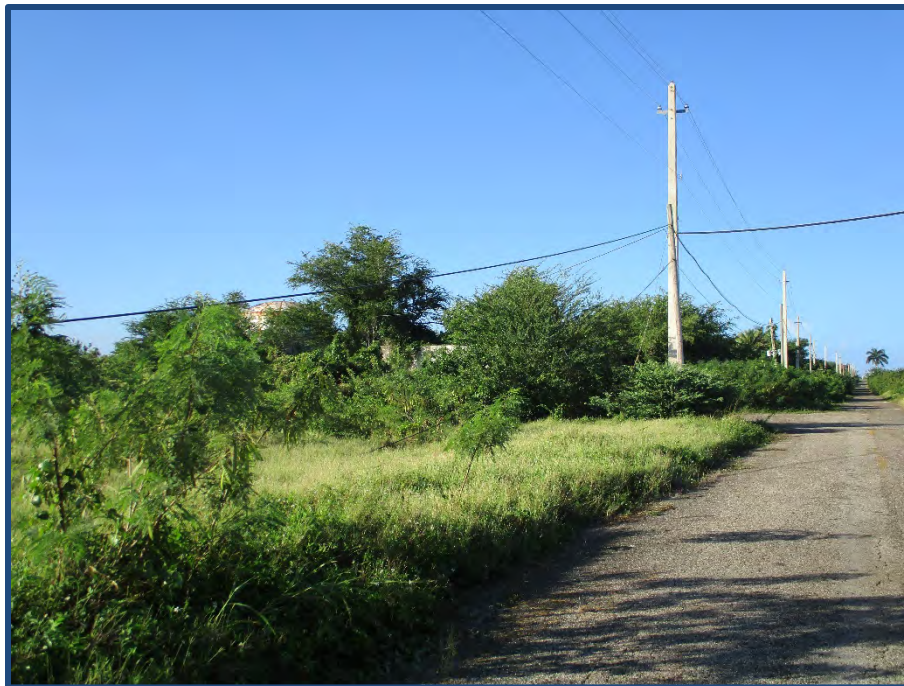
Photo 5.2-7: Overgrown locations with damaged utility risk, facing south.
