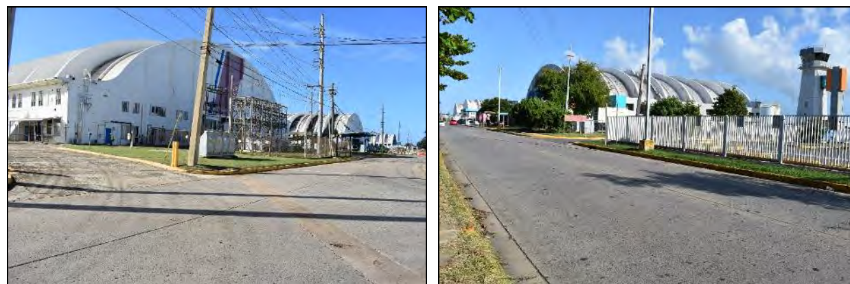
9 Photo 6.1-324, left Control Tower, Hangar 5, modern FedEx hangar, Hangar 3, and Hangar 2 (left to right); Photo 6.1- 10 325, right, Hangar 3 with Hangar 2 at far right.
