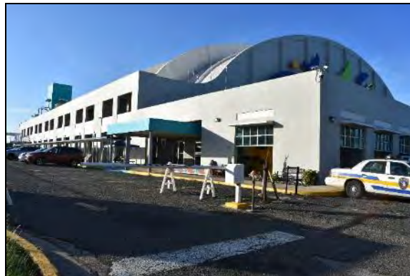
1 Photo 6.1-296 Hangar 5: E side and N street-side elevations.
