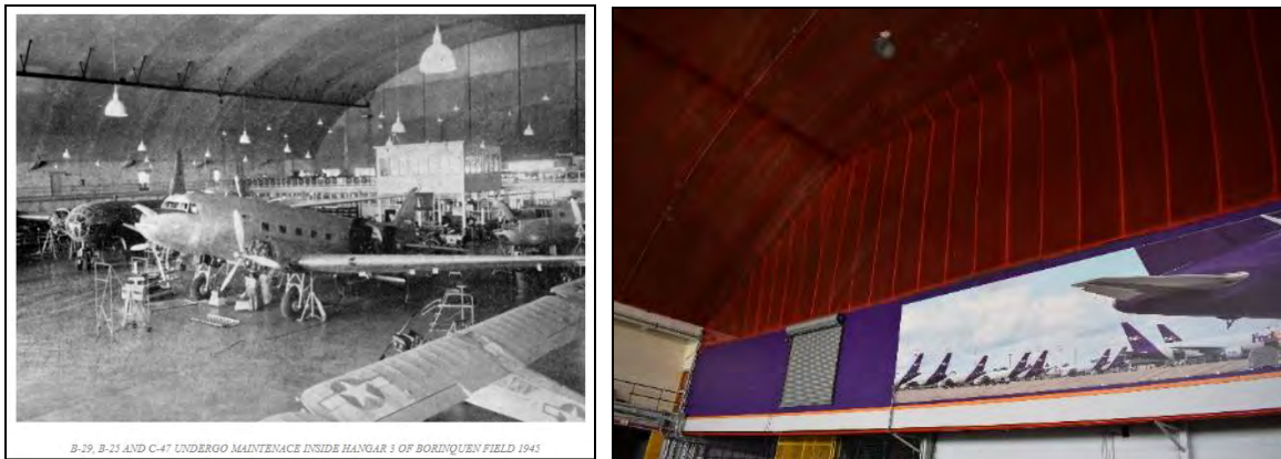
14 Hangar 3: Photo 6.1-286, left, looking northwest at hangar interior in 1945 (source: RFBHA 2015b); Photo 6.1-287, 15 right, looking northwest at north wall and roof; note that wall, roof, and hanging light supports beneath mesh continue 16 to look those in the 1945 image.
