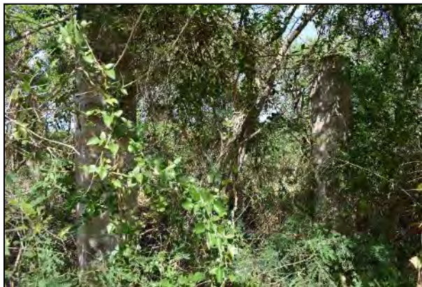
3 Photo 6.1-354 Gazebo: concrete-block posts
