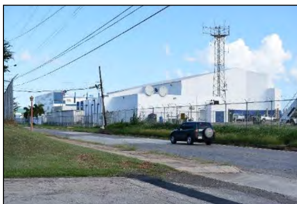
3 Photo 6.1-462 Building 575 (Hangar): north rear and west side elevations
