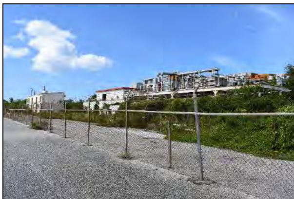
11 Building 1129 (Armaments and Electrical Shop): Photo 6.1-388, south front elevation with Boiler Building at left.
