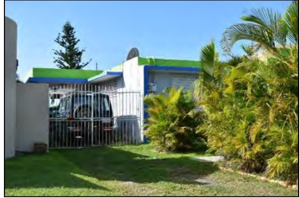
4 Photo 6.1-135 131 Loop Street
