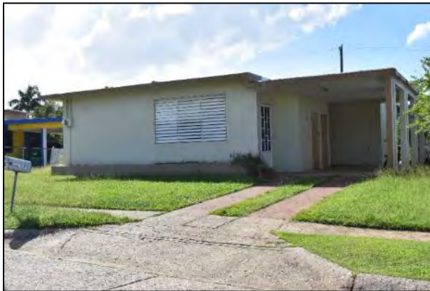
2 Photo 6.1-67 107 Lighthouse Drive
