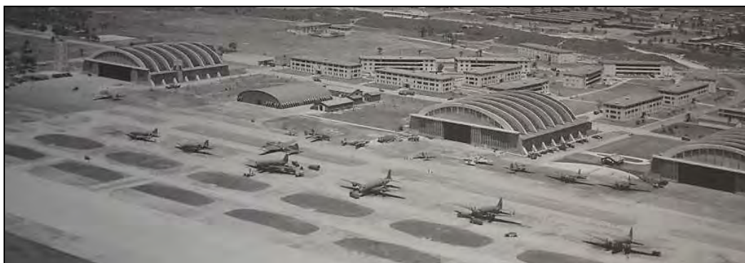
4 Photo 6.1-329 Borinquen Field with Control Tower and Hangar 5 at far left, Building 404x and Hangar 3 at center, and 5 Hangar 2 at far right in 1943.
