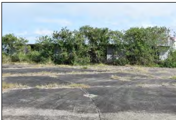
6 Photo 6.1-357 Building 1104 (Storage and Supply): west front elevation
