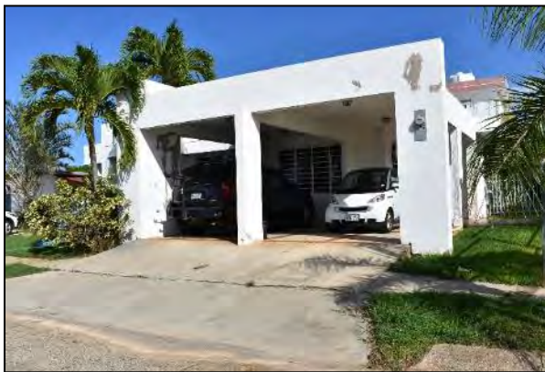
4 Photo 6.1-128 124 Loop Street
