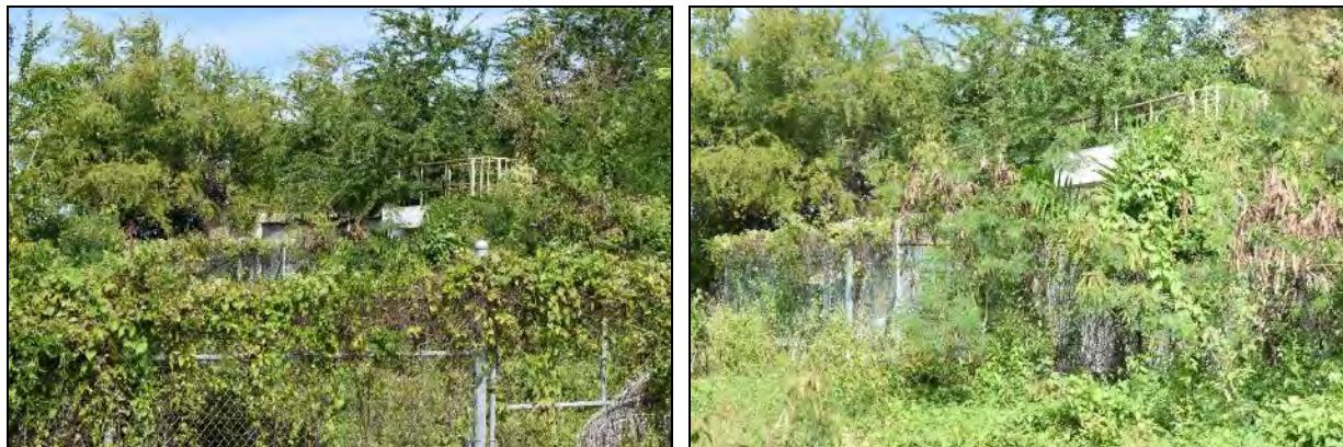
6 Water Storage Building: Photo 6.1-371, left, north elevation; west side and south front elevations; Photo 6.1-372, right, 7 north elevation framed by chain-link fencing.
