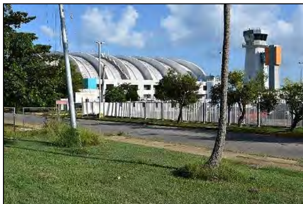
3 Photo 6.1-328 Hangar 5 and Control Tower
