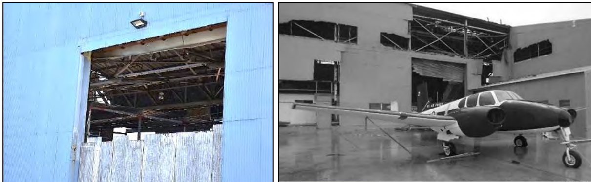
1 Building 572 (Hangar): Photo 6.1-448, left, damage an interior at bay west of nose bay; Photo 6.1-449, right, September 2 2017 view, post-Hurricane Maria (source: View From the Tower , October 1, 2017).
