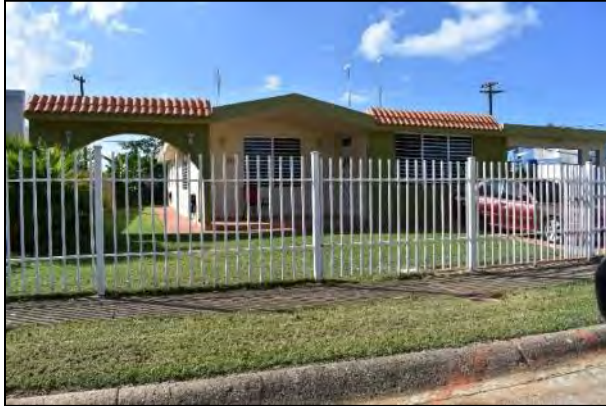
1 Photo 6.1-89 129 Lighthouse Drive
