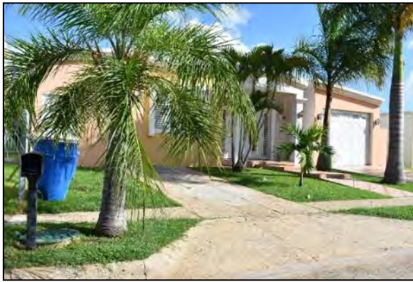
2 Photo 6.1-126 122 Loop Street
