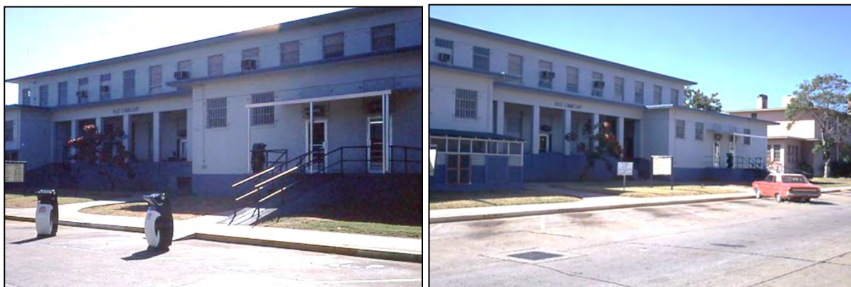
6 Building 506 (Commissary): Photos 6.1-200-201, north front elevation, 1972-1973 (source: 7 https://rameyafb.wordpress.com/2010/11/13/pictures-of-ramey-afb-puerto-rico/ ).
