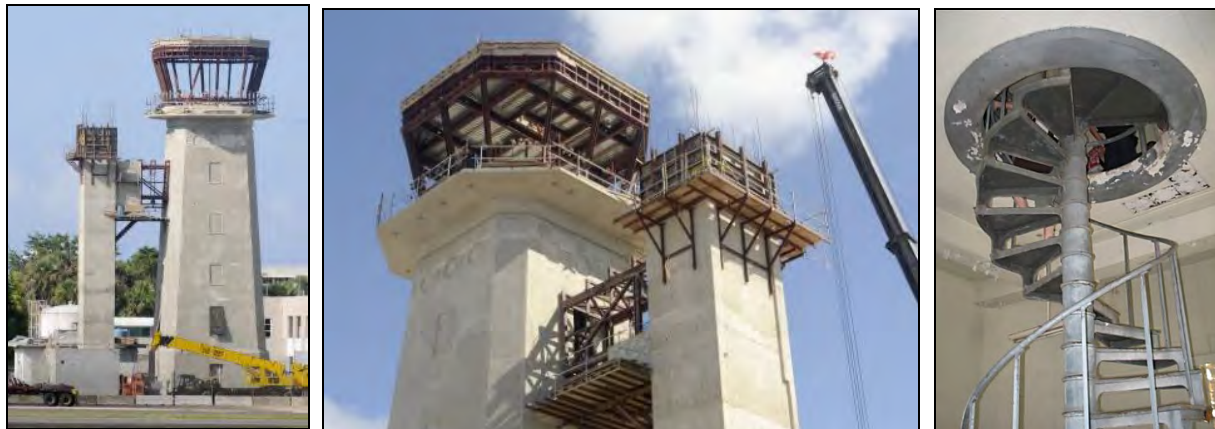
11 Control Tower: Photo 6.1-308 (left) and Photo 6.1-309 (center), new elevator shaft and cab just after hoisting into place, 12 2015 (source: http://rameyafb.net/category/blog/page/11/ ); Photo 6.1-310, right, circular stair in 2009 (source: 13 https://www.facebook.com/photo.php?fbid=1108193270675&set=q.137328899312&type=1&theater&ifg=1 ).
