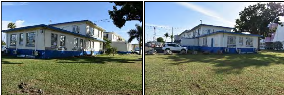
3 Building 406 (Fire Station): Photo 6.1-231, left, south front and west side elevations; Photo 6.1-232, right, west side 4 and north rear elevations.
