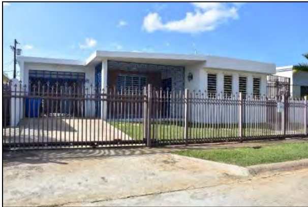
2 Photo 6.1-85 125 Lighthouse Drive
