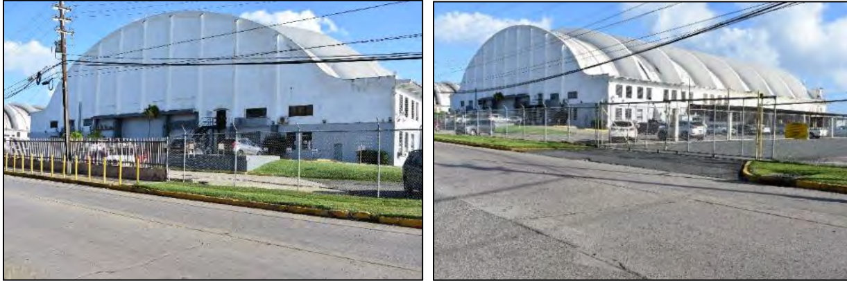
1 Hangar 3: Photo 6.1-284, left, north street-side and W side elevations; Photo 6.1-285, right, north street-side and west 2 side elevations, note intact bays at side elevation.
