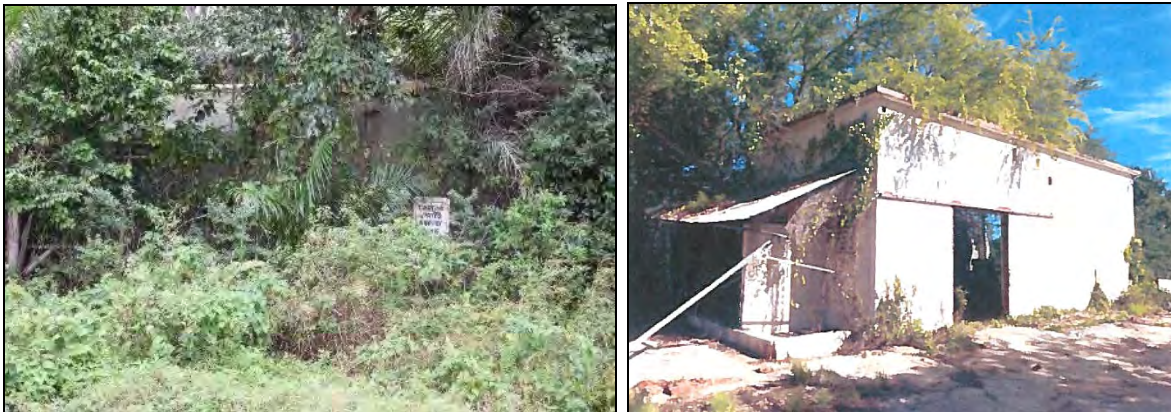
9 Building 1133 (Captive Water Supply Tank Building): Photo 6.1-367, left, north rear elevation with gray water tank; 10 Photo 6.1-368, right, west side and south front elevations (source: AM Group 2018:98).
