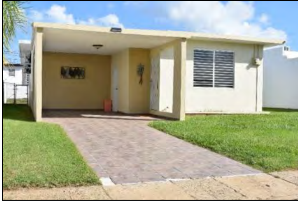
1 Photo 6.1-124 120 Loop Street
