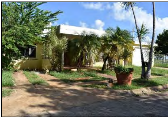
4 Photo 6.1-110 102 Loop Street
