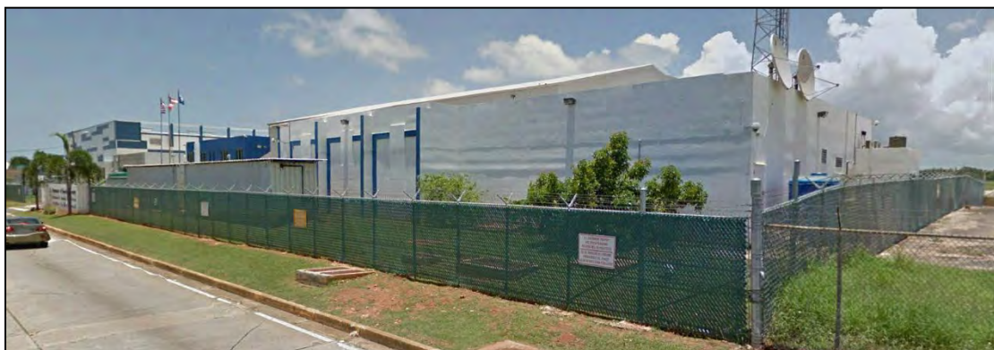
15 Photo 6.1-459 Building 575 (Nose Dock Hangar): Google Earth aerial of north front and west side elevations of Building 16 575 at right and new associated hangar at left, 2019.
