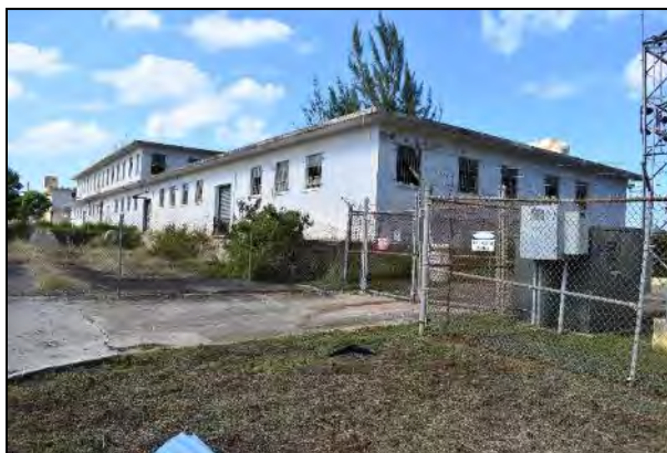
5 Photo 6.1-199, Building 506 (Commissary): south rear and east side elevations.
