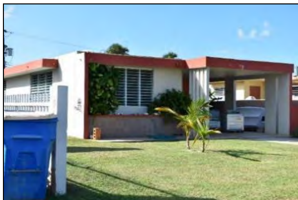
1 Photo 6.1-23 Largely intact houses: 119 Loop Street 2 Avenue
