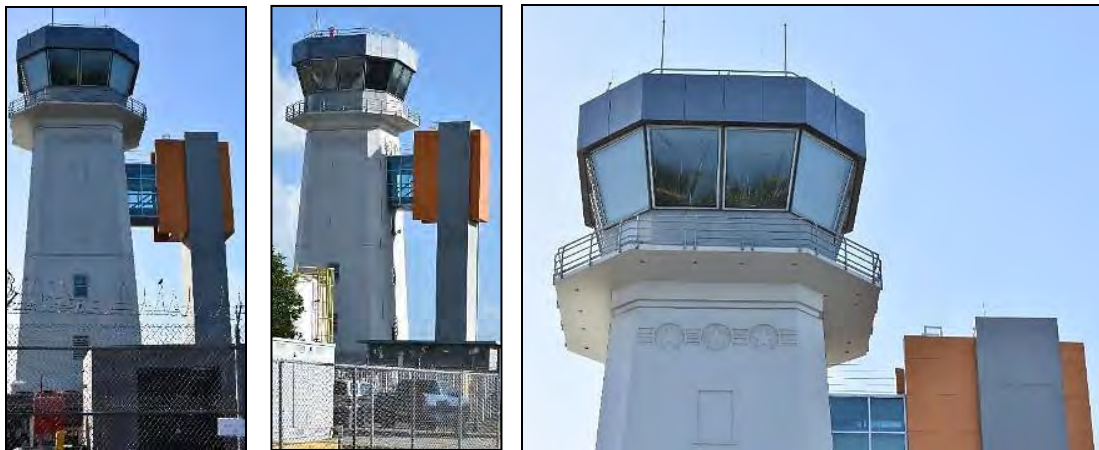
1 Photos 6.1-311 – 6.1-313, Control Tower: views looking S at tower, with concrete walls, form and insignia intact and 2 2015-added cab, elevator tower, and connector.
