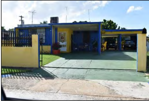
1 Photo 6.1-65 105 Lighthouse Drive
