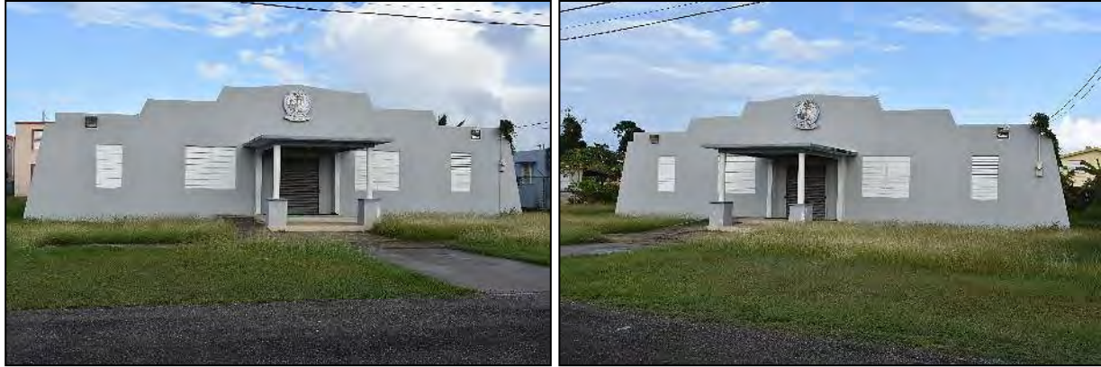
1 Photos 6.1-499 (left) and Photo 6.1-500 (right) Paul Revere Lodge No. 98: W front elevation.
