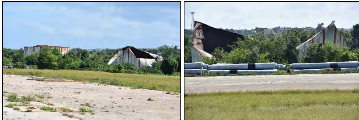
1 Tank 1214 (Fuel Storage Tank): Photo 6.1-474, left, looking southeast at Tanks 1215 and 1214, left to right; Photo 6.1- 2 475, right, looking south at Tank 1214.
