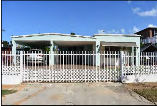
1 Photo 6.1-112 106 Loop Street
