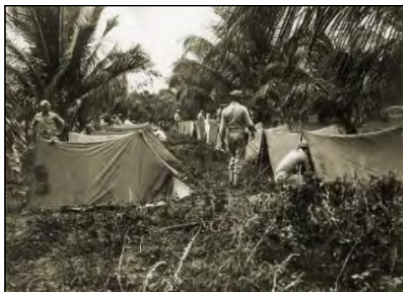
8 Photo 3.3-1 "Base housing" in 1939 (source: RAFBHA 2015a).
